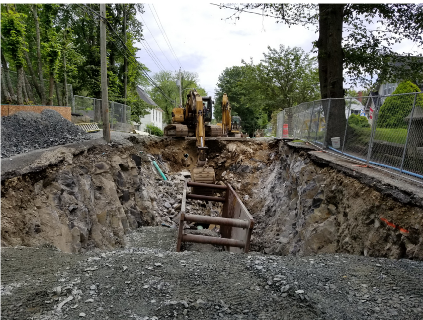
An excavator prepares for pipe laying up the hill on School Street. Work crews encountered much rock in this area.
