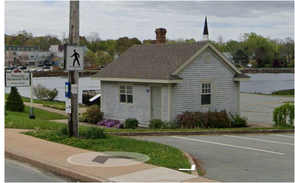
Lane’s Lift Station
