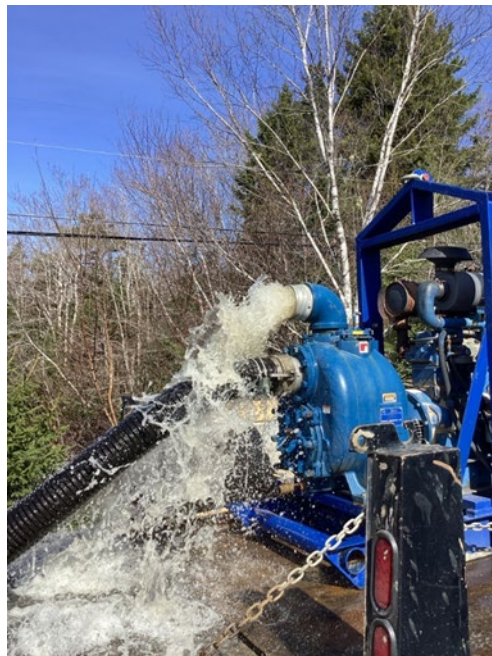
Figure 1. Flow testing a dry hydrant
