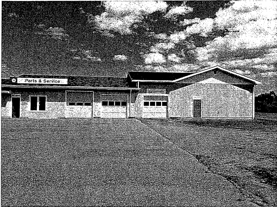
Photo 5 - Western side of the Site building with three (3) service bays (location of TP9).
