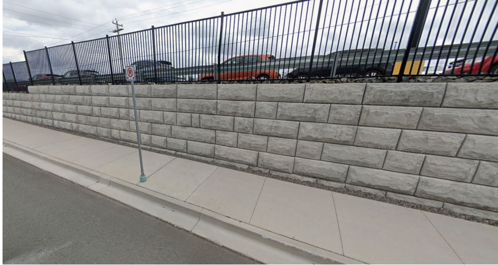
Figure 2. Example of gravity retaining wall blocks completed at Cape Breton Regional Hospital.
