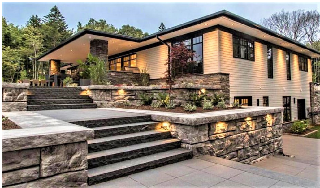
Figure 3. Example of stairs constructed using gravity retaining wall blocks.
