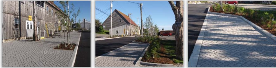
Permeable Pavers in Hawthorne Street, Yarmouth (Source: CBCL Design)
