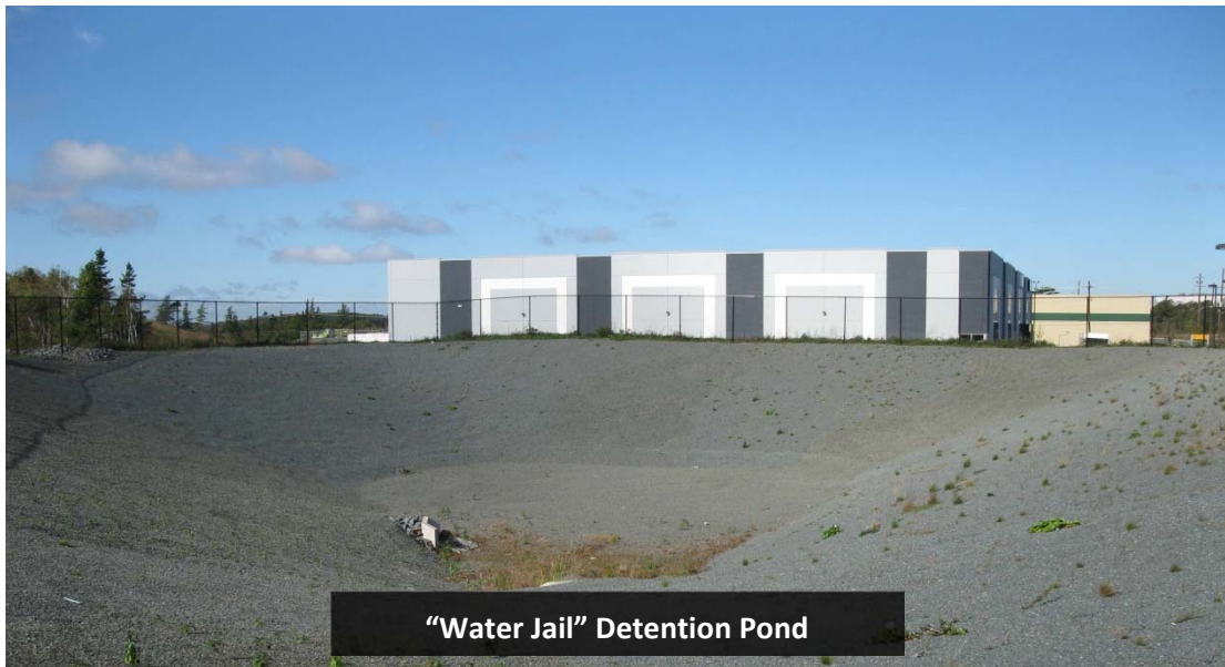
Example of Halifax Water "Red Book" Dry Detention Pond in Burnside (Source: CBCL Design)
