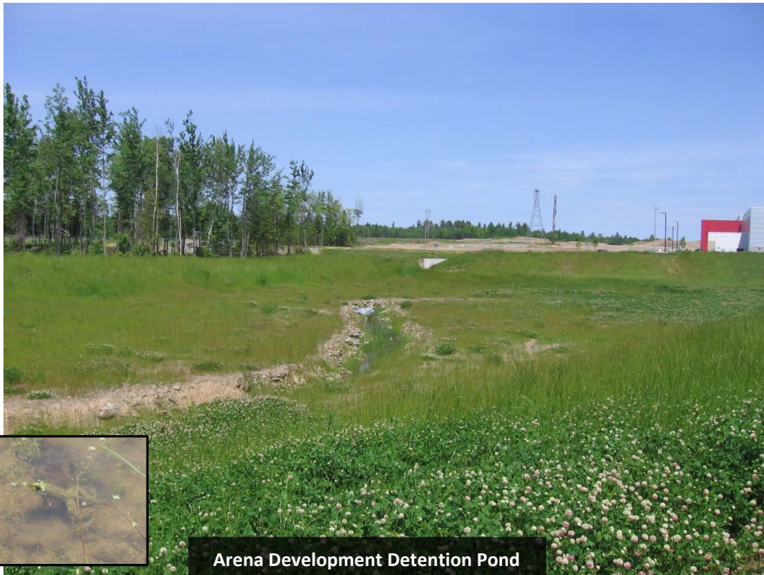
Example of Dry Detention Pond in Fredericton (Source: CBCL Design)
