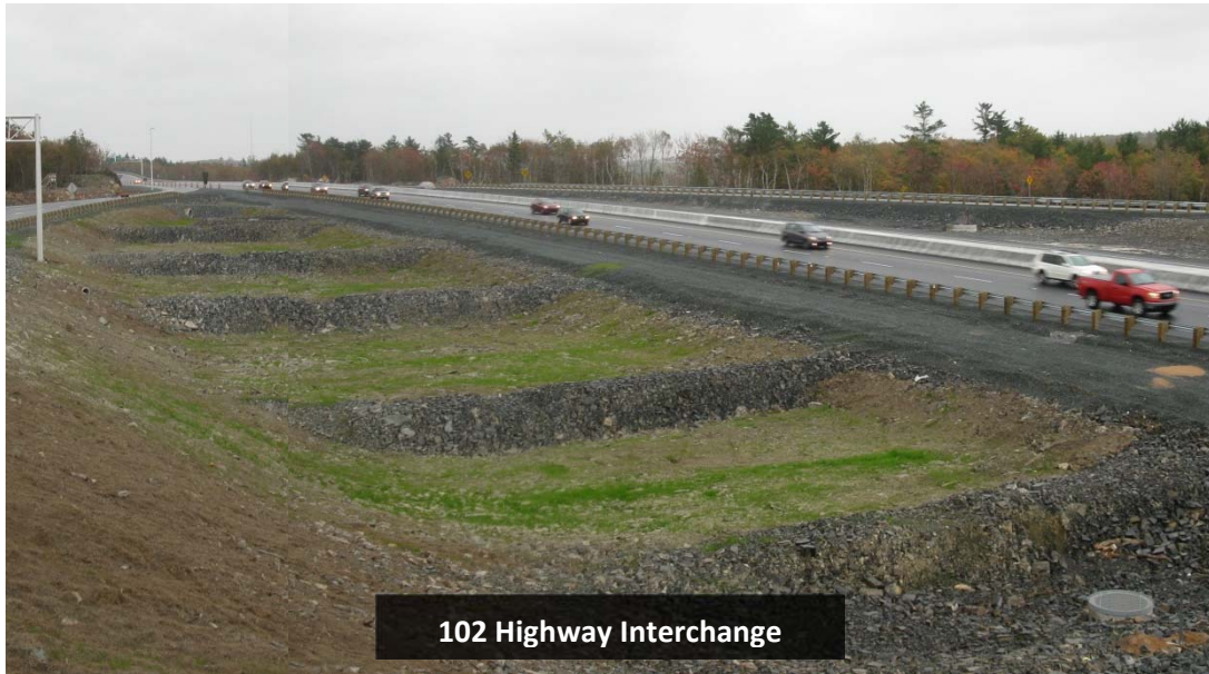
Enhanced Grass Swales (Source: CBCL Design)
