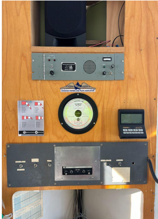
Photo of the Aircraft Communication System in the Terminal Building.
