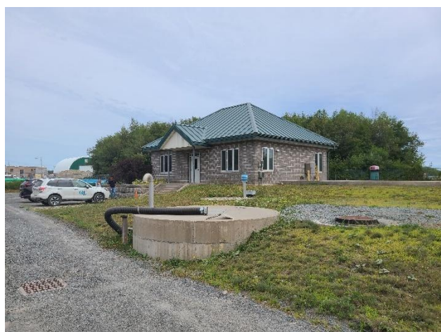
Septage Receiving Station
