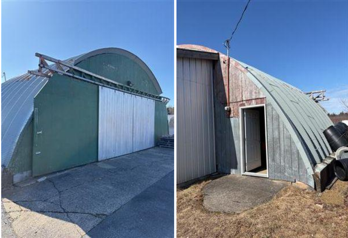
Photo of Hangar B from the airside (left) and groundside (right).
