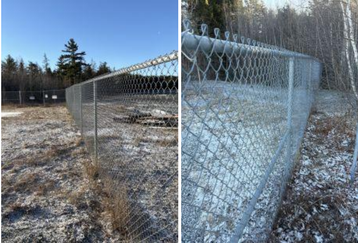
Photo of Fencing from the groundside.
