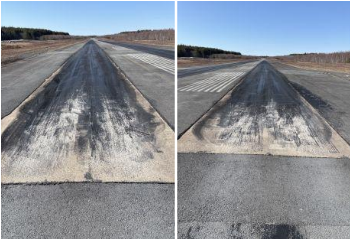
Photo of Burn Out Pads from Airside.
