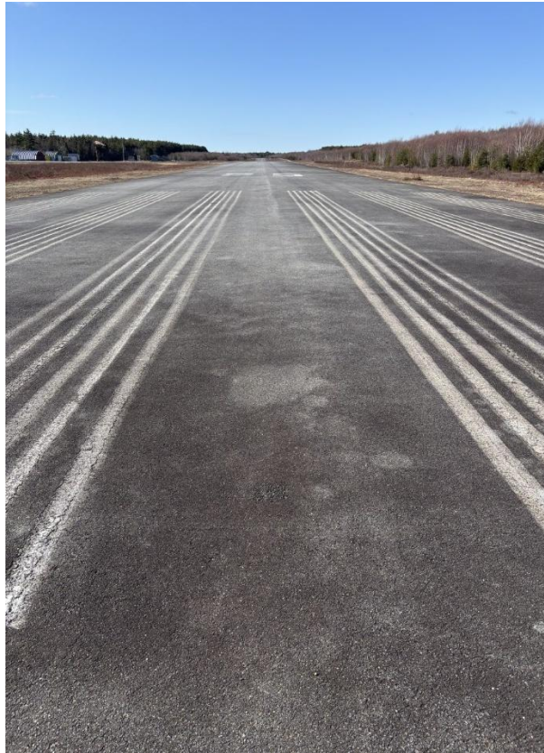
Photo of Runway from the airside.
