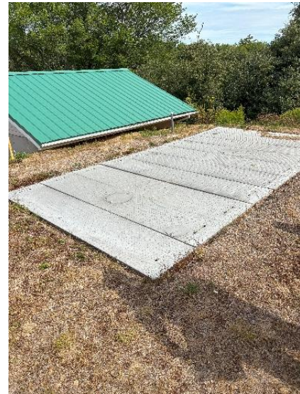
Sludge Holding Tank
