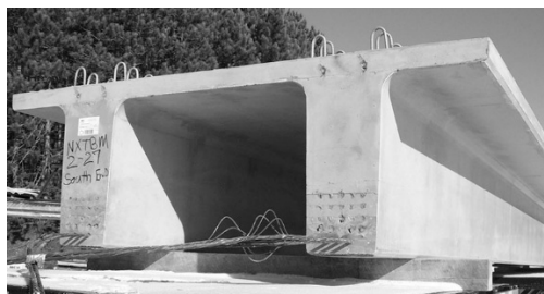
Figure 5 - Northeastern Extreme Bulb Tee Girder (PCI.org)
