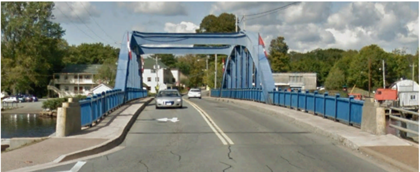
Figure 2 - Existing bridge roadway and active transit lanes
