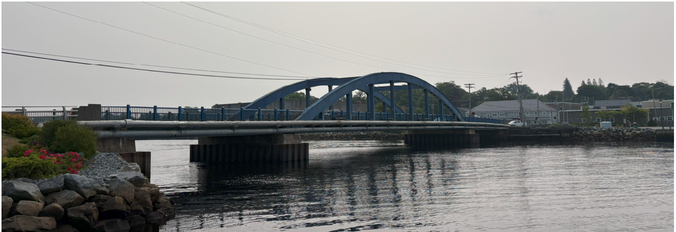
Figure 1 - Existing bridge elevation view
