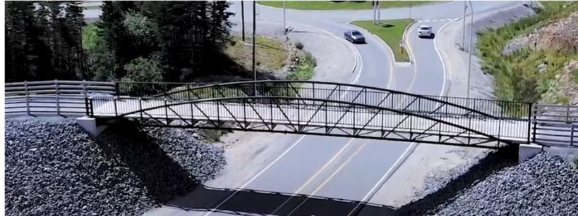
Figure 6 - Example of Prefabricated Bowstring Bridge Option (Algonquin, 2020)
