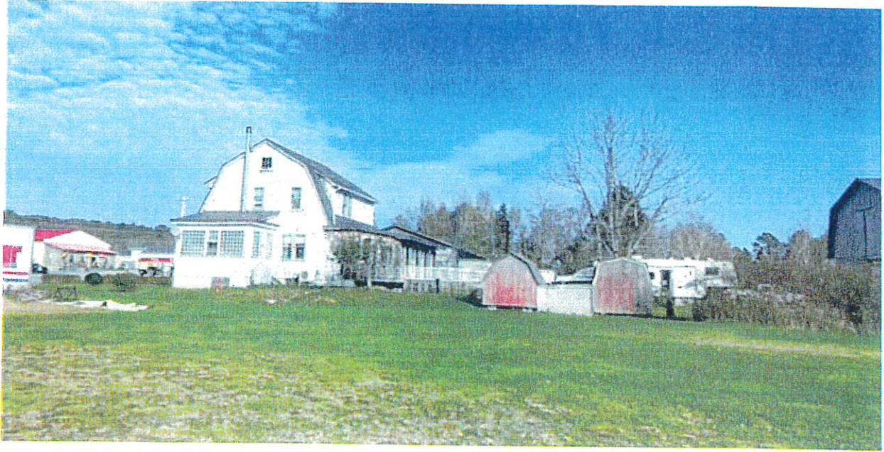
Ground view of buildings over the survey line
