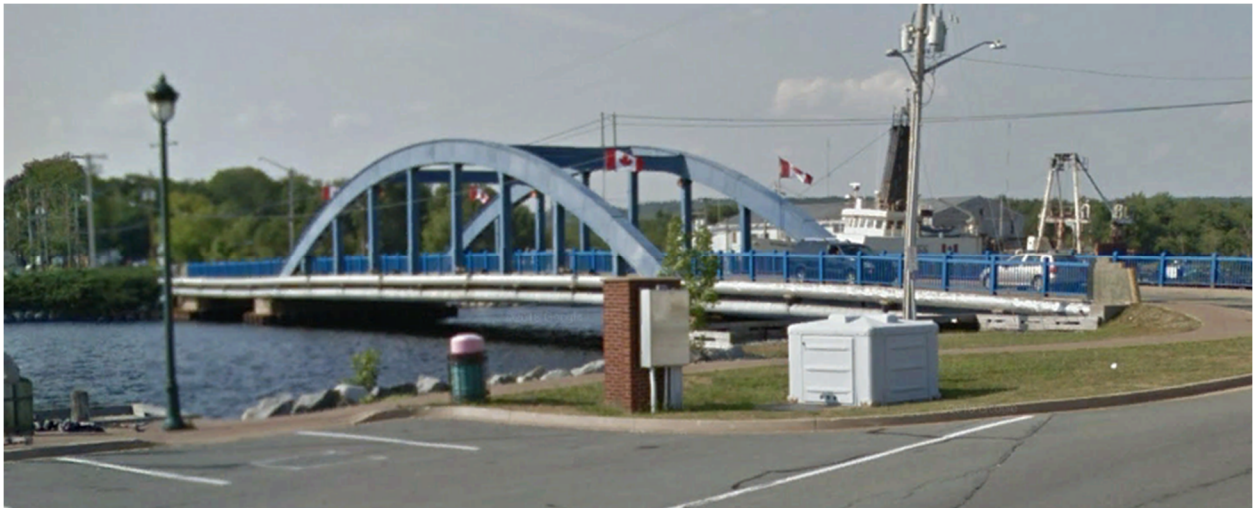
Figure 3: West side of the bridge showing the existing force main
