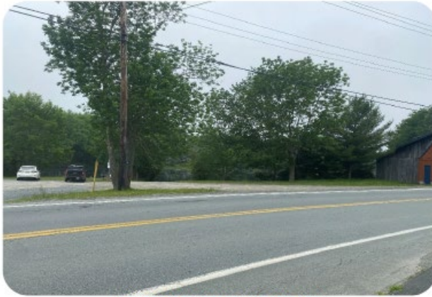
HIGHWAY #8 FRONTAGE – LOOKING WEST
