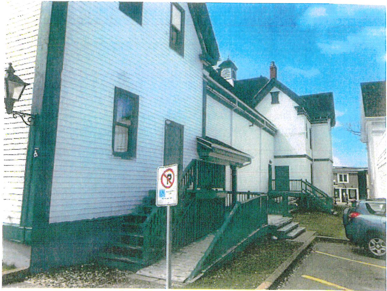
East Side of Building. View from rear parking lot.
